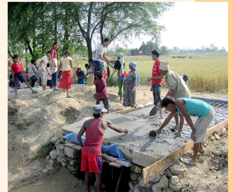
Communities constructing culvert in Binauna VDC, Banke
